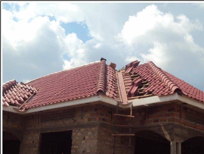
Above: One of the client housing using concrete roof tiles
