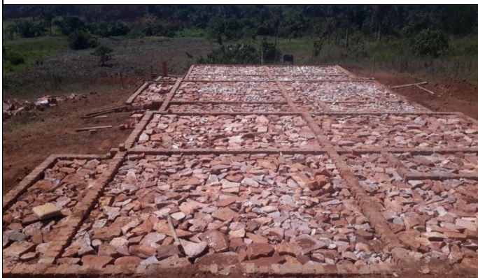
Incomplete 3units slab
